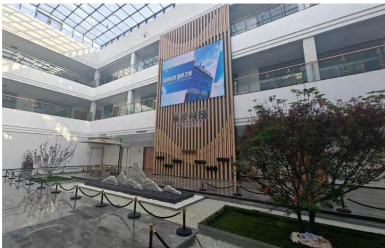
Natural Lighting Design of the Office Building at the Ordos Manufacturing Base
