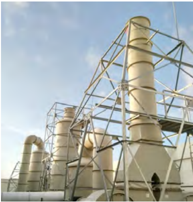
晶澳基地废气净化塔 Exhaust gas purification tower at JA Solar's manufacturing base
