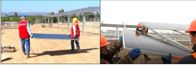
Figure 2. The size and weight of 182mm Wafer Size Module basically reach the upper limit of convenient handling and installation by two persons.
