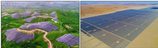
Figure 4. Single support length is limited in case of serious terrain undulation, but ultra-long supports can be available for flat terrain.
