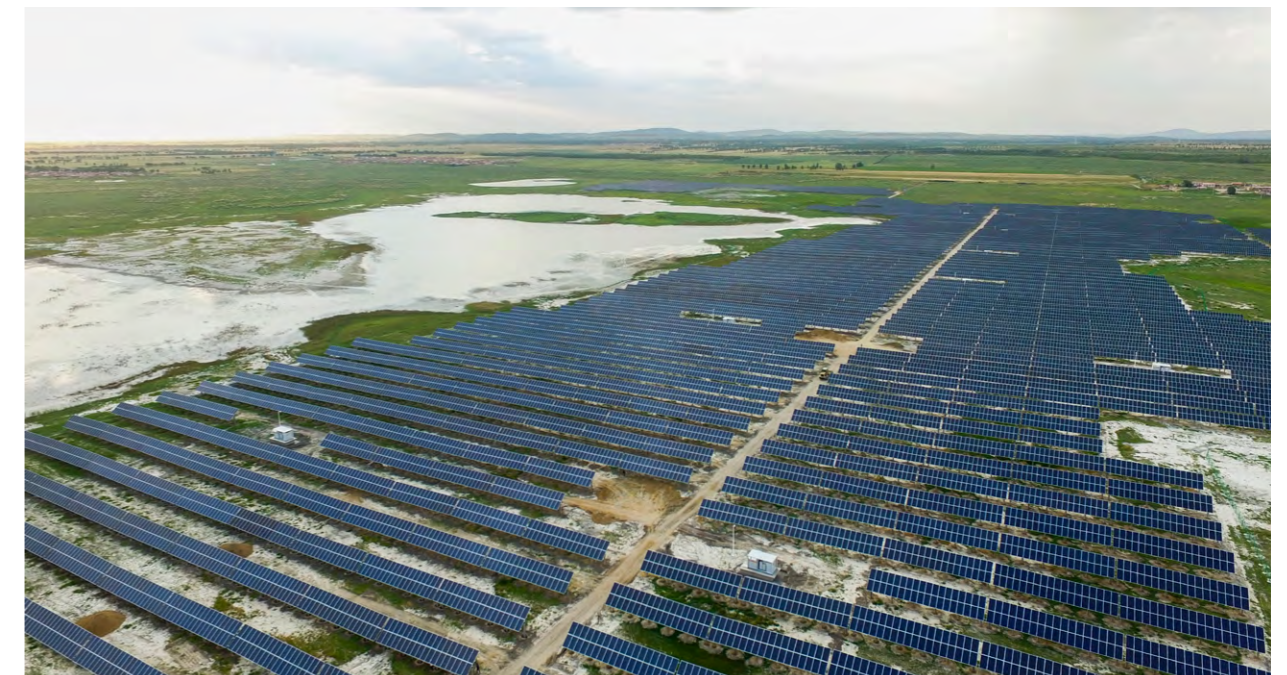
晶澳河北康保20MW光伏扶贫电站 JA Solar's photovoltaic poverty alleviation power station in Kangbao, Hebei Province (20MW)
