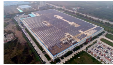
邢台基地厂房分布式项目 Plant Distributed Project in Xingtai Manufacturing Base
