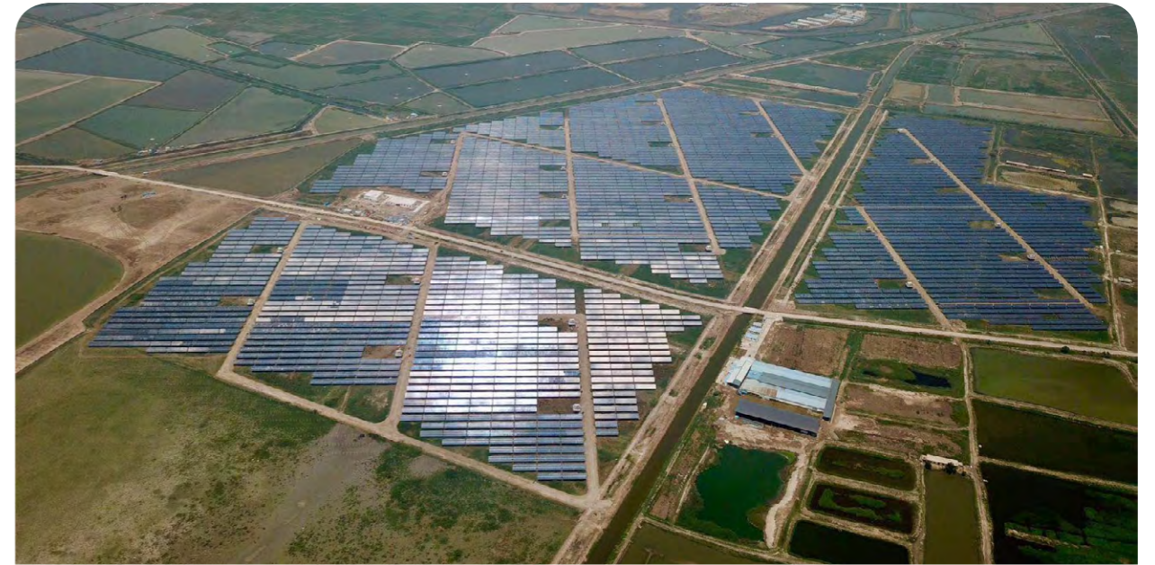
晶澳宁夏贺兰30MW光伏电站 JA Solar's 30MW Photovoltaic Power Plant in Helan, Ningxia
