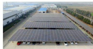
东海基地车棚分布式项目 Carport Distributed Project in Donghai Manufacturing Base
