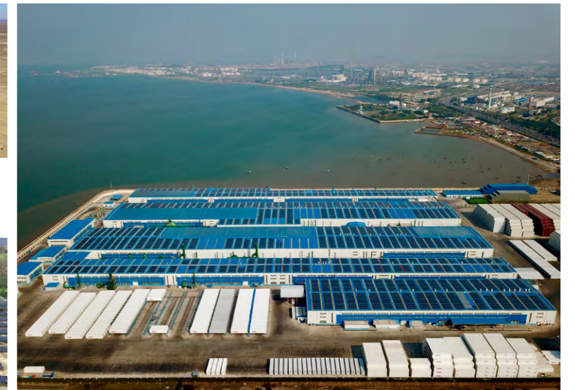
晶澳青岛太平货柜分布式电站 JA Solar's Taiping Container Distributed Photovoltaic Power Plant in Qingdao
